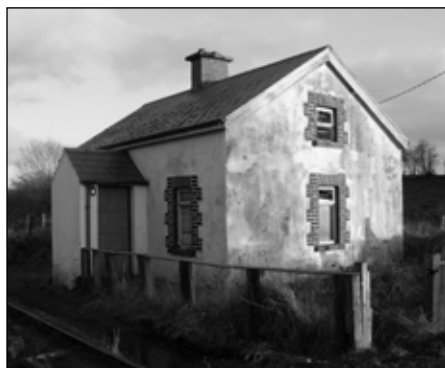
Level-crossing Gate House
