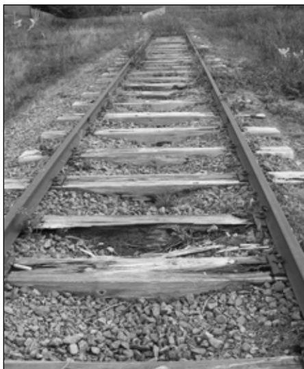
Cleared Track Between Collooney and Coolaney
