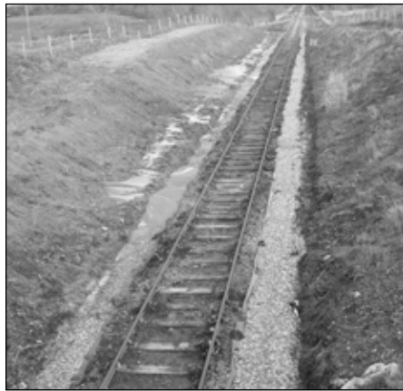
Cleared Track West of Charlestown
