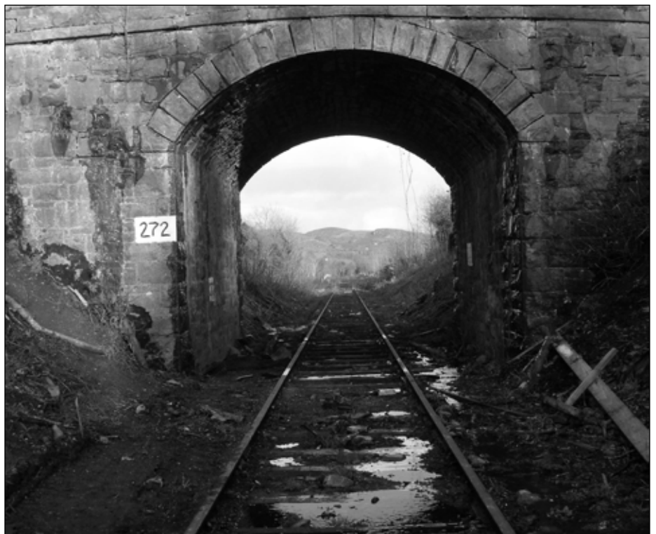
Bridge No 272, east of Coolaney
