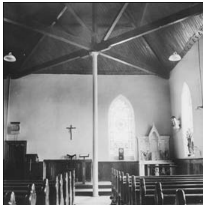
Photo 1: Looking up the interior of the Men's House, Keash R.C. Church, Co. Sligo, as it was prior to the start of renovations in 1977.
