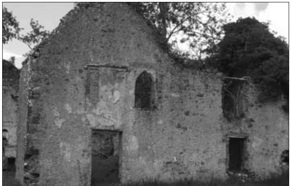
This is a photograph of the ruin of Templehouse Castle today, showing the Jacobean window which was blocked up in the 18th century when render was applied to the whole façade covering the red brick. The underlying seventeenth century red brick mansion is probably unique in this part of the country and possibly in Ireland as a whole. Photograph: John Coleman.
